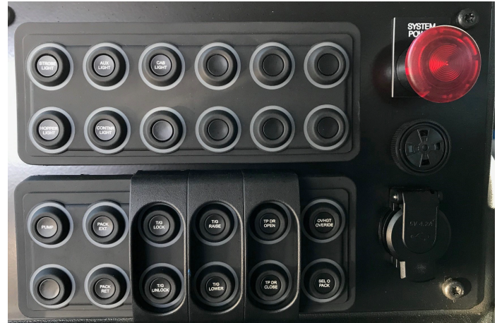
Figure 54. In-Cab Main Control Panel
