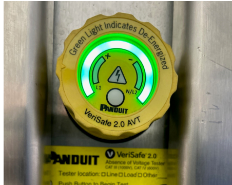
Figure 43. Absence Tester: After Pressing Circular Button the Outer Ring Turns Green if Body Electrical System is De-Energized
