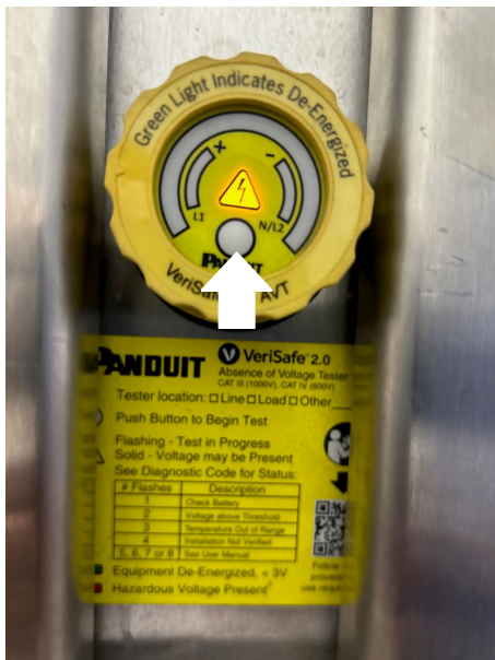
Figure 17. Absence Tester: Pressing Circular Button (White Arrow) Initializes Testing (Flashing Triangle Hazard Symbol)
