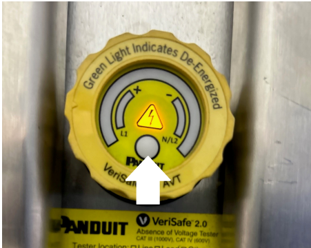
Figure 42. Absence Tester: Pressing Circular Button (White Arrow) Initializes Testing (Flashing Triangle Hazard Symbol)
