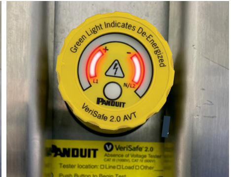
Figure 44. Absence Tester: After Pressing Circular Button the Two Inner Rings Turn Red if When Voltage is Detected
