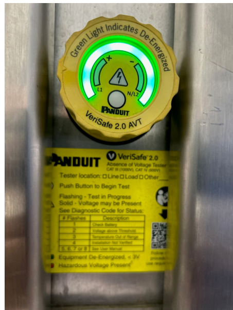
Figure 18. Absence Tester: After Pressing Circular Button the Outer Ring Turns Green if Body Electrical System is De-Energized
