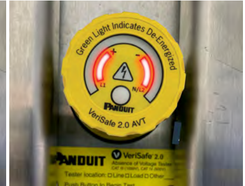
Figure 46. Absence Tester: After Pressing Circular Button the Two Inner Rings Turn Red if When Voltage is Detected
