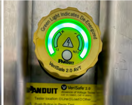
Figure 45. Absence Tester: After Pressing Circular Button the Outer Ring Turns Green if Body Electrical System is De-Energized
