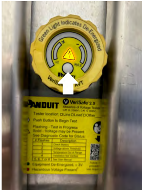
Figure 19. Absence Tester: Pressing Circular Button (White Arrow) Initializes Testing (Flashing Triangle Hazard Symbol)
