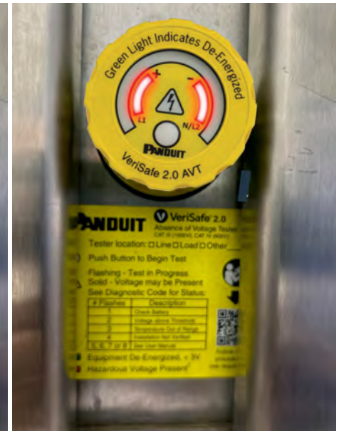
Figure 21. Absence Tester: After Pressing Circular Button the Two Inner Rings Turn Red if When Voltage is Detected
