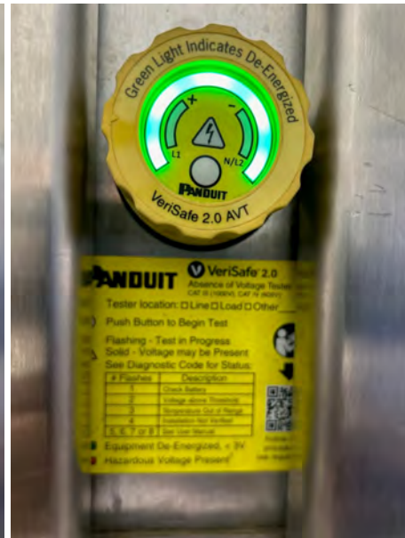
Figure 20. Absence Tester: After Pressing Circular Button the Outer Ring Turns Green if Body Electrical System is De-Energized
