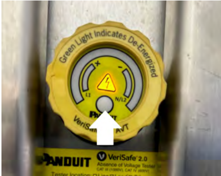
Figure 44. Absence Tester: Pressing Circular Button (White Arrow) Initializes Testing (Flashing Triangle Hazard Symbol)
