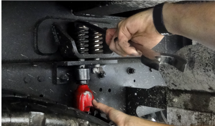
Figure 47. Removing Bolts and Springs from Chassis Mounting Brackets
